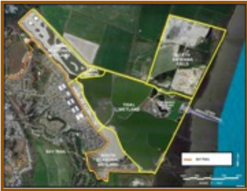
Hamilton Field's restoration includes land inundated by seasonal flooding, U.S. Army Corps of Engineers photo
