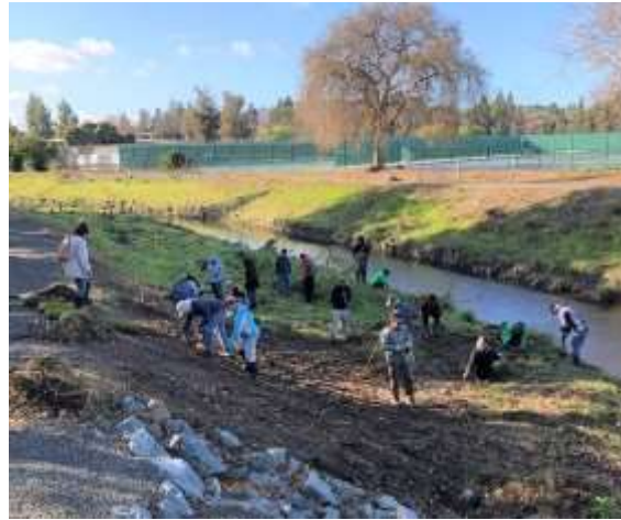
Grayson Creek restoration Golf Club Road bridge in Pleasant Hill
