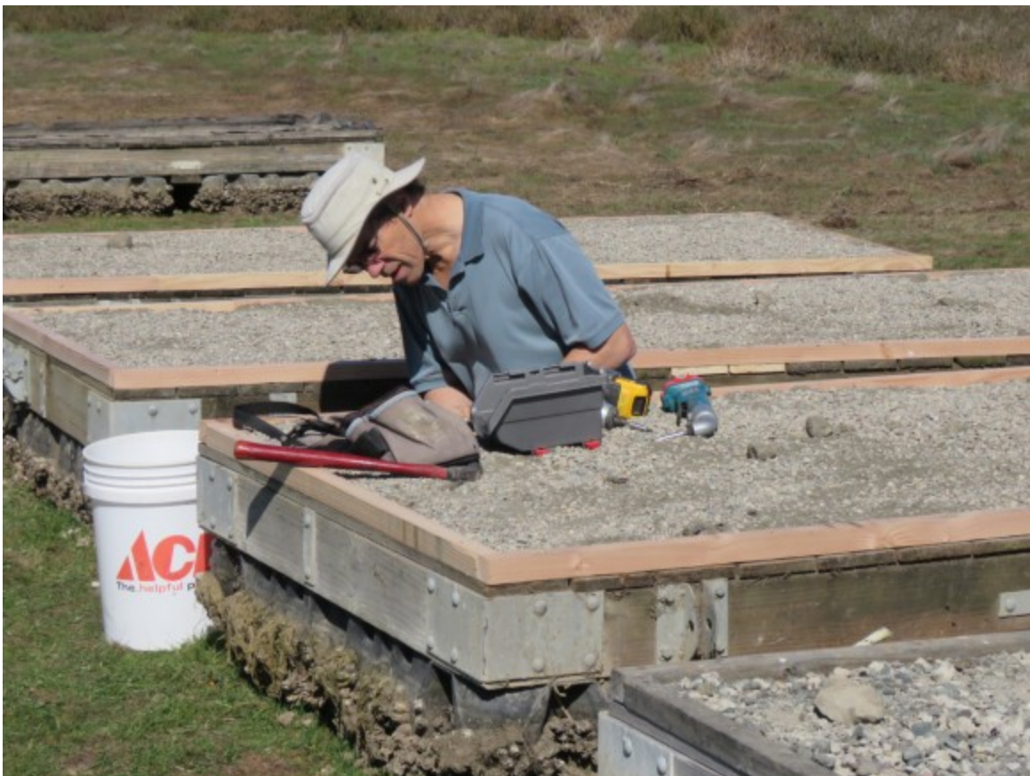
Alan Bade repairs a nesting raft McNabney Marsh
