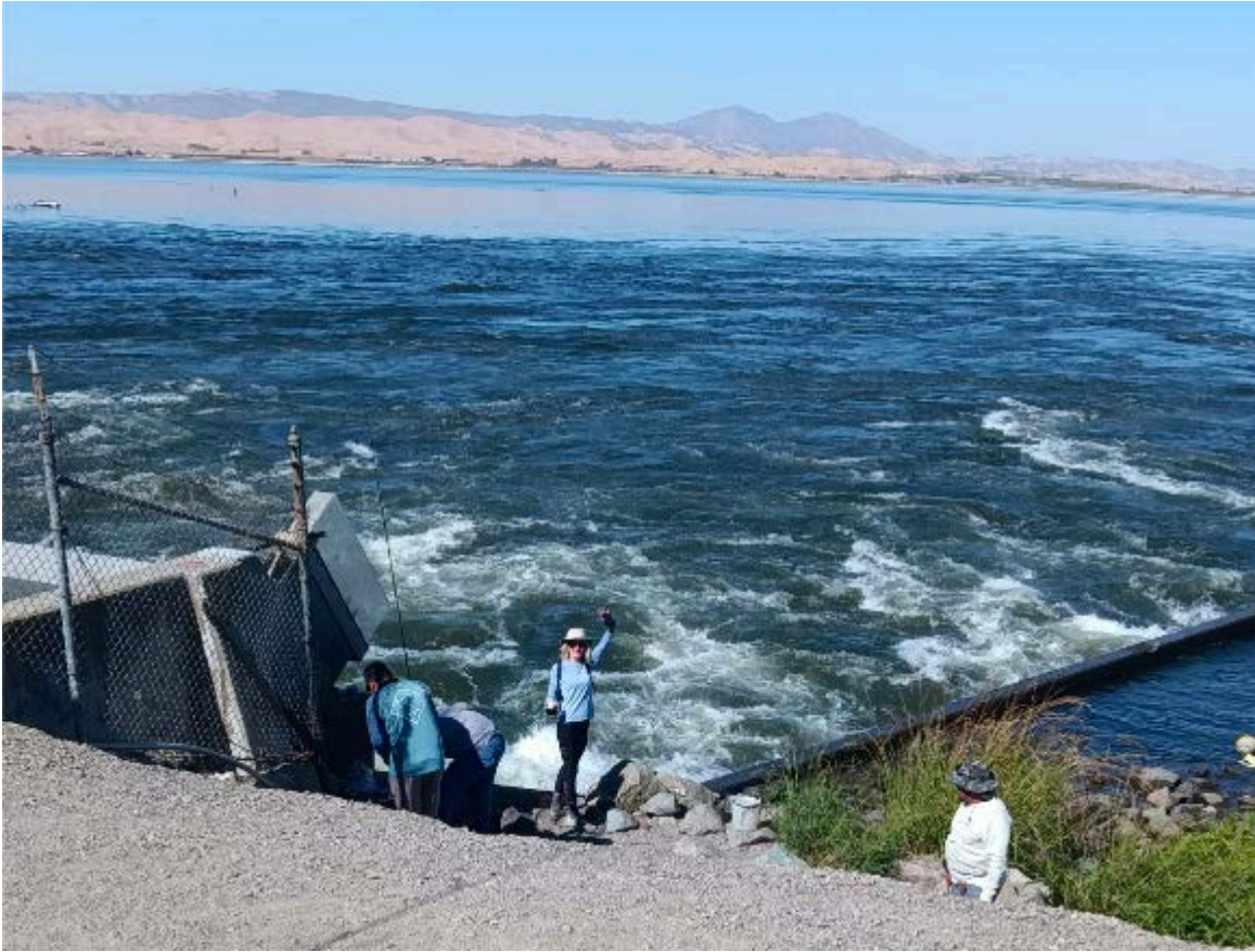
MDBA Secretary Karin Deas inspecting the intake gates at Clifton Court Forebay, where water from the delta is stored and ultimately sent south via the California Aqueduct.
